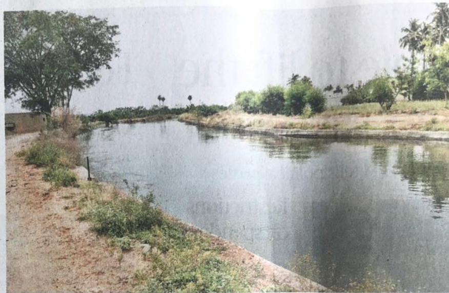
The Kalingarayan Canal in Erode. ■ M. GOVARTHAN
